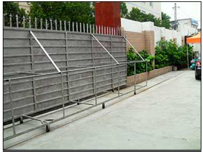
Not enough lamps at fence lines
