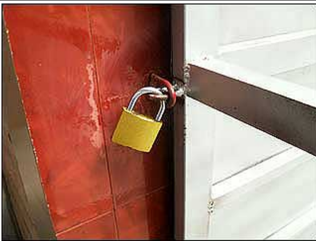
Factory gate lock
