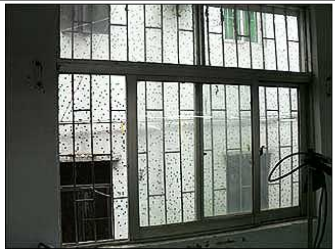
Metal grills on outside of windows
